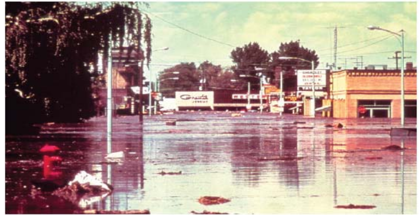
FIGURE 1.3 Teton Dam failure. Flood waters advancing through Rexburg, Idaho. SOURCE: BOR.
